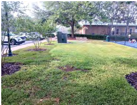
Clubhouse boat ramp area- install sod on two fertilizer burnt sections of turf. WARRANTY WORK. Photo below.
